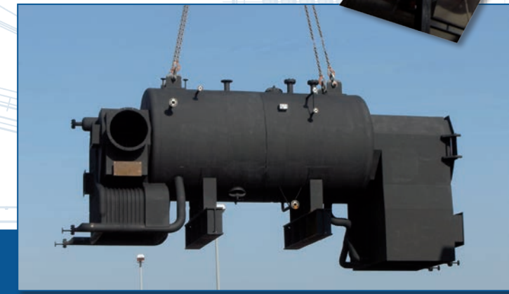
Installation of a superheated steam boiler
